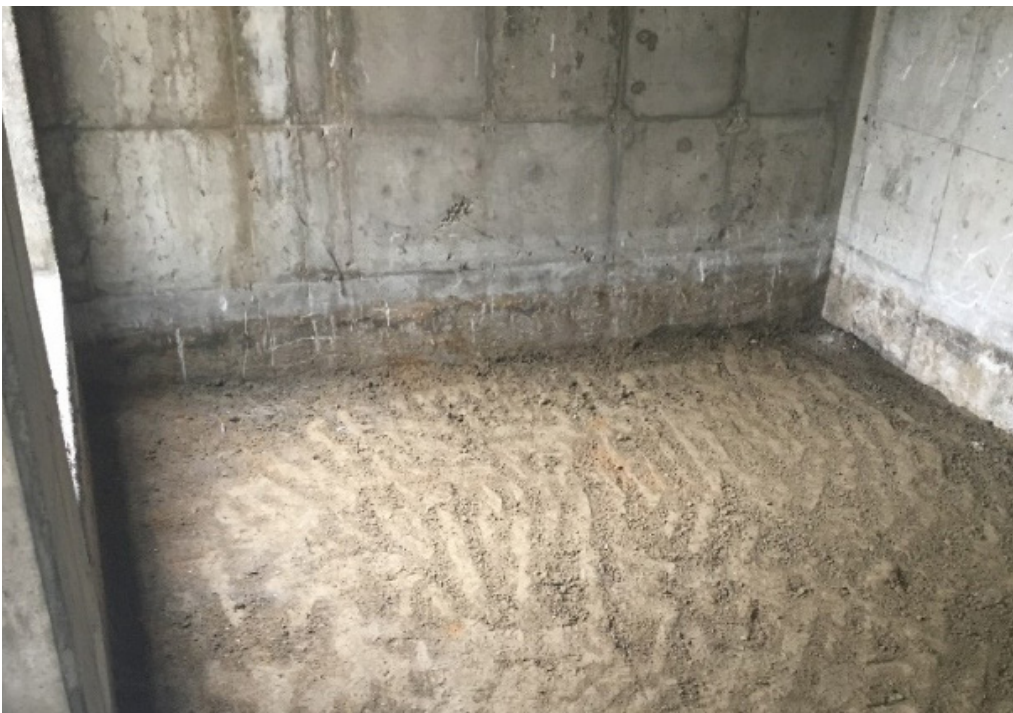
The vault after remediation was completed.
